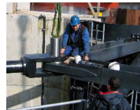
Hydraulic system solution for driving and controlling the rotating sector gates of the New Harbor lock in Bremerhaven – from planning and design to production and installation.
